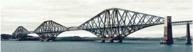
Fig. 1.2 – Baker and Fowler's Firth of Forth Railway Bridge. The two main spans are each 1700 feet long. Opened 1890.
