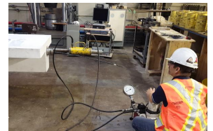
Fig. 35.2 – Skilled worker post-tensioning cables in a concrete member using a hydraulic jack.
