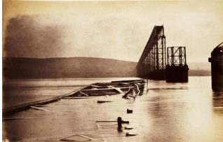
Fig. 16.2 – Firth of Tay Bridge, 29 December 1879. The engineer, Sir Thomas Bouch, was unable to produce the wind calculations during the subsequent investigation.
