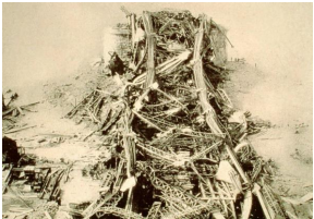
Fig. 1.4 – Cooper's Quebec Bridge after collapse.
